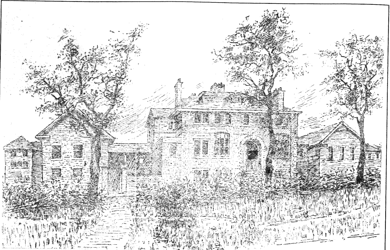
The stone facade of Kettering General Hospital in Rothwell Road, illustrated by local artist, poet and hairdresser, George Harrison, to celebrate the opening of the building in the autumn of 1897.
